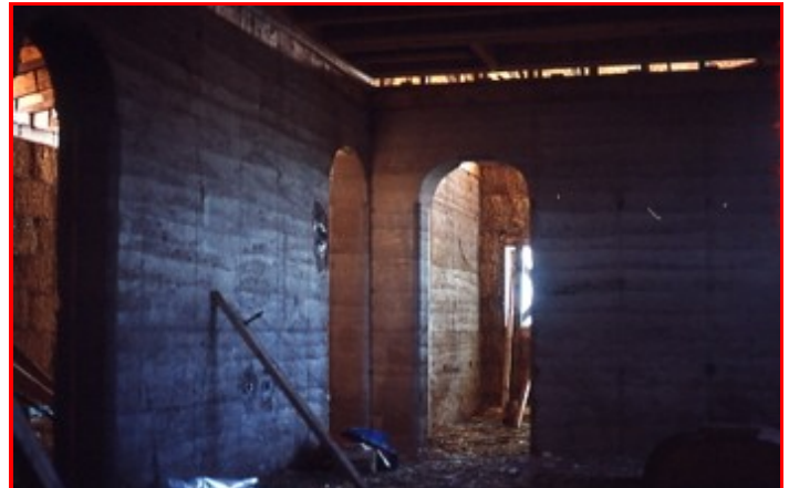
81: Alberta rammed earth construction, ASH-Inc.
