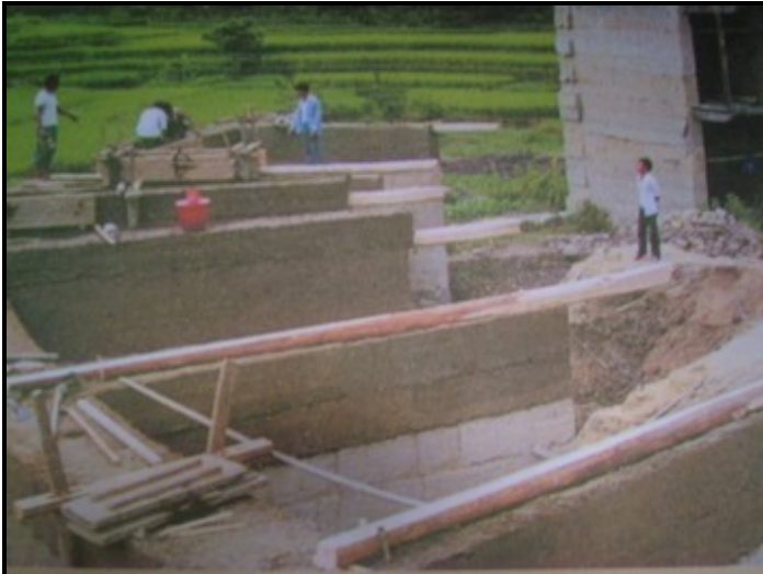
78: Hakka rammed earth walls, Zhenfu museum
