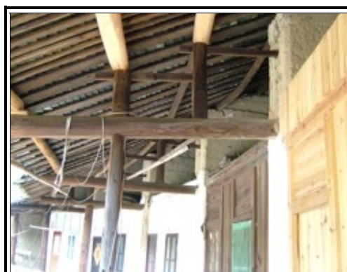
5: structural/wall upgrade, Chaoyang
