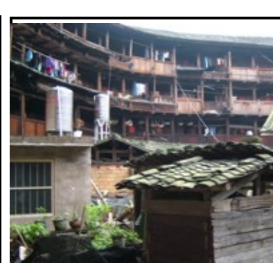
19: DHW tanks, Shuncheng
