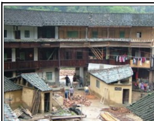
4: repair (Chaoyang, Hongkeng)
