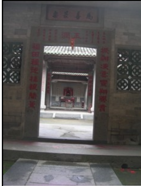
118: entry, courtyard Ancestral Hall
