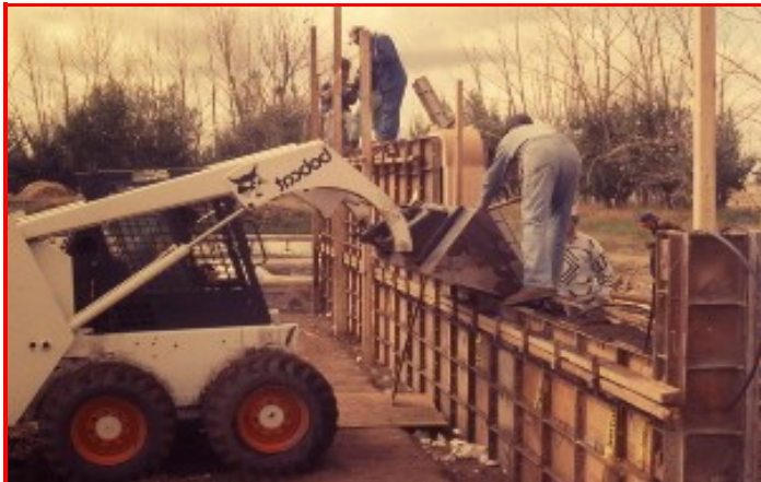
80: rammed earth construction, 1990, ASH-Inc.
