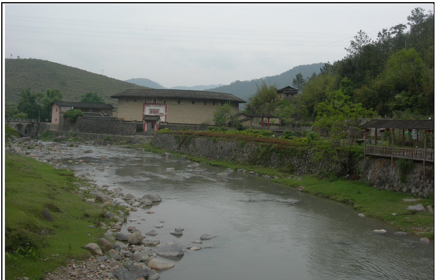
1: Zhenfu Lou, on Nanxi River is a stand-alone tulou, with row house, gardens & ecotourist facilities
